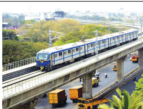
Chennai Metro Rail Limited (CMRL)
