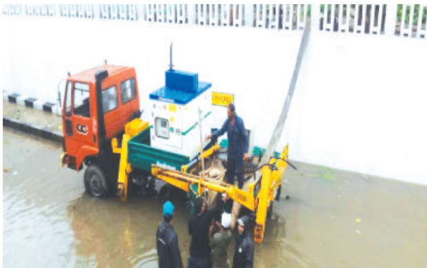
Pump set deployed in subways
